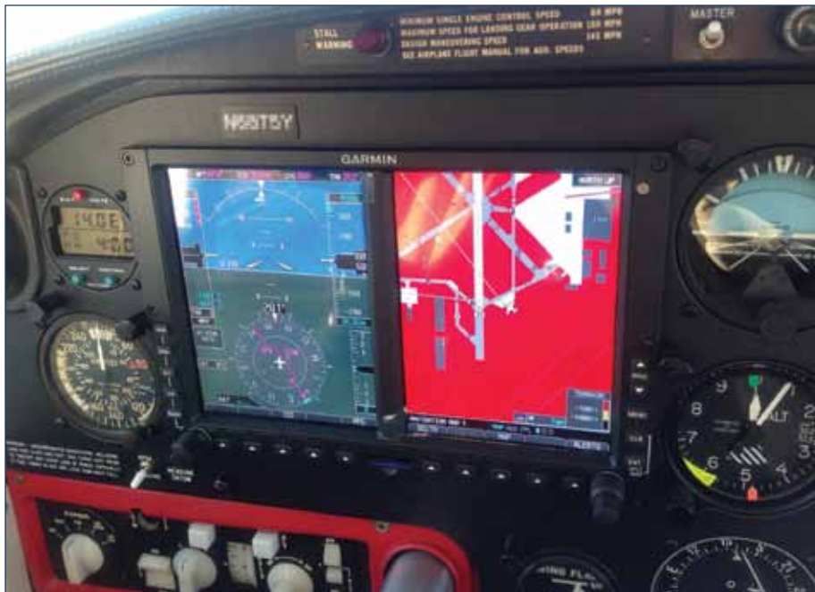
Garmin G500 installed in an Aztec panel, original autopilot at lower left.
